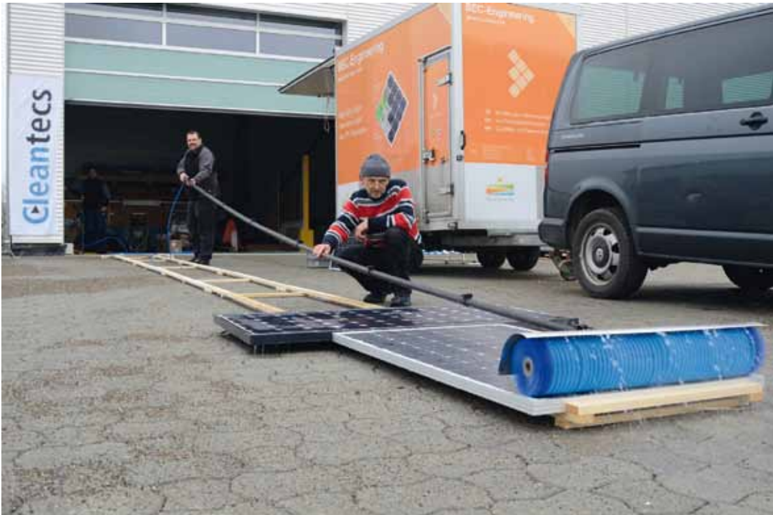
Image 1: Presentation of the module cleaning process with the C700 cleaning device
