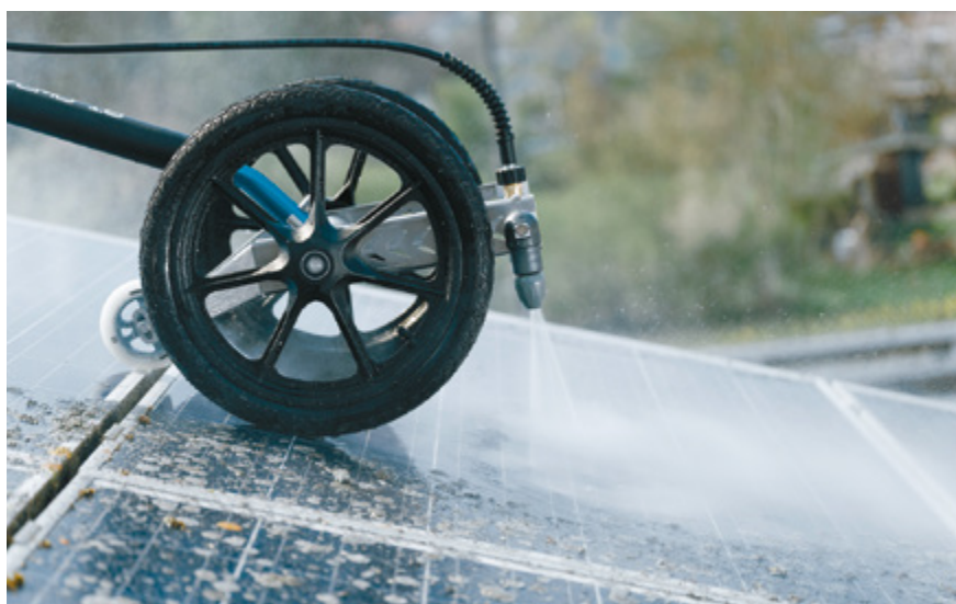
Lichens are always a huge problem for solar systems.
